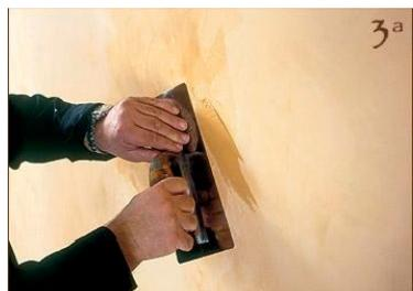
Step 7 - At this point the product will penetrate into every little crack and with slight pressure the surface will be perfectly smooth. We apply... and remove Spatula Stuhhi for about 1 square meter and ...
